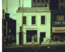
1 building 330 king street front view
