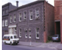
1 langdon building king street melbourne front view
