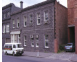
1 langdon building king street melbourne front view
