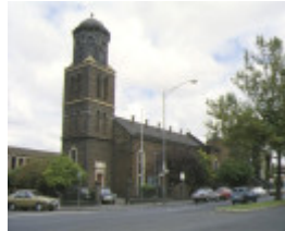
1 st james old cathedral king street melb external view
