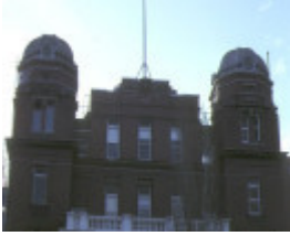
pre 1994 former queen victoria hospital lonsdale street melbourne roof dooms detail jul1984
