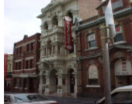
sum kum lee little bourke street melbourne front view jul1999
