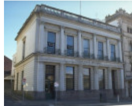
H00109 photo former union bank lydiard st ballarat
