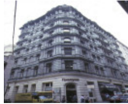
stalbridge chambers little collins street melbourne front elevation may1989
