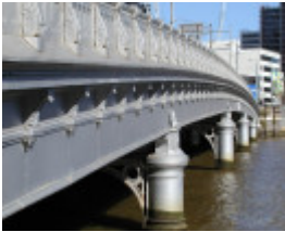
h01448 queens bridge queensbridge street over yarra river melbourne close view
