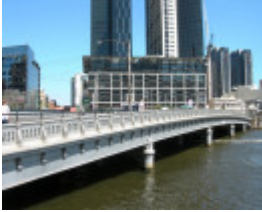
QUEENS BRIDGE SOHE 2008
