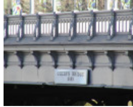
h01448 queens bridge queensbridge street over yarra river melbourne detail view
