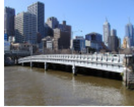
h01448 queens bridge queensbridge street over yarra river melbourne distant view
