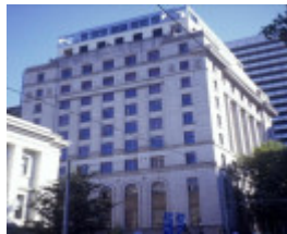
h00965 former port of melbourne authority building exterior she project 2003
