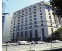
former port of melbourne authority building market street melbourne side view mar1980
