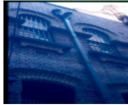
h00473 warehouses niagara lane2
