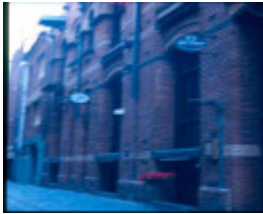
h00473 warehouses niagara lane3
