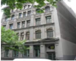
LOMBARD BUILDING SOHE 2008
