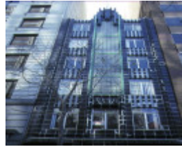
1 alkira house queen street melb front view
