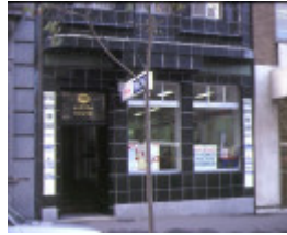
alkira house queen street melb detail shop front jul1984
