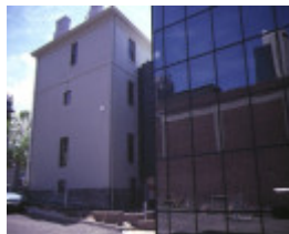
former residence queen street melbourne rear view jan1985
