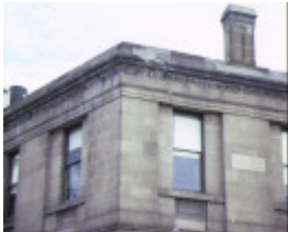
bank of nsw queen street melb roof detail
