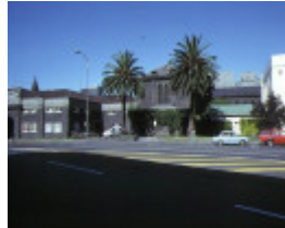
1 old melbourne gaol russell street melbourne front view jan1979
