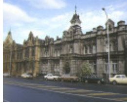
1 city watch house russell street melbourne front view 1993
