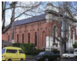
1 former church of christ stanton street abbotsford general view sep1985
