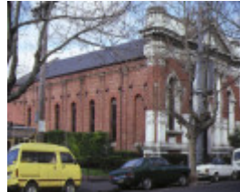
1 former church of christ stanton street abbotsford general view sep1985
