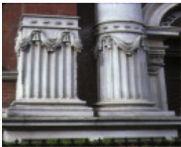
former church of christ stanton street abbotsford facade detail sep1985
