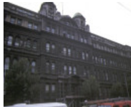
1 former victorian railway headquarters spencer street melbourne vline head office
