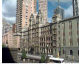
hotel windsor spring street melbourne front elevation
