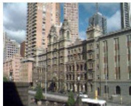
hotel windsor spring street melbourne front elevation
