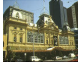
1 princess theatre spring street melbourne front view after restoration
