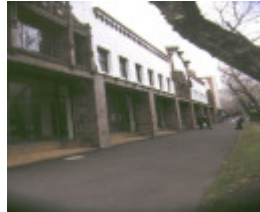
former kellow falkiner showrooms st kilda road melbourne street view
