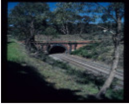
ELPHINSTONE RAILWAY TUNNEL
