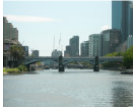
PRINCES BRIDGE SOHE 2008
