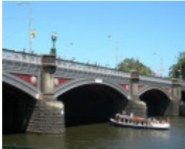
PRINCES BRIDGE SOHE 2008
