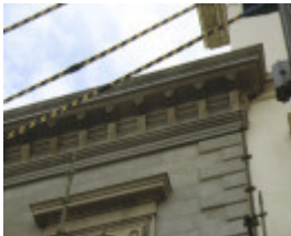
anz bank ballarat roof detail
