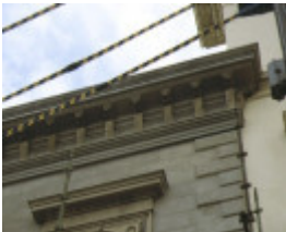
anz bank ballarat roof detail
