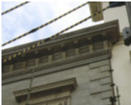
anz bank ballarat roof detail
