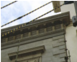
anz bank ballarat roof detail
