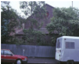
horticultural hall victoria street melbourne rear view 1991
