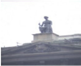
1 library of the supreme court william street melbourne pediment
