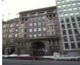
queensland building william street melbourne front view may1978
