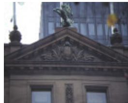
scottish house william street melbourne roof design jul1985
