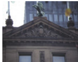
scottish house william street melbourne roof design jul1985
