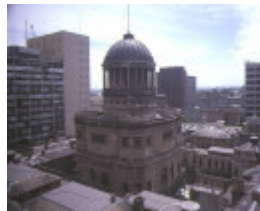
law courts william street melbourne tower view feb1985
