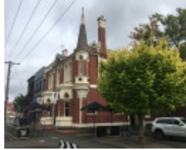
Corner Sturt Street Errard Street
