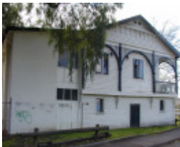
h00682 melbourne university boat club shed yarra bank off jeffries pde melbourne other side she project 2004
