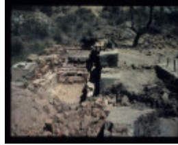
MORNING LIGHT MINE EXCAVATION
