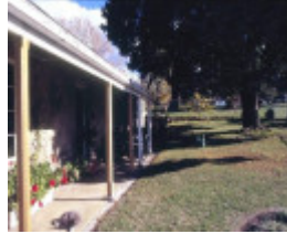
h00318 stratford lodge coliban park rd metcalfe verandah she project 2003
