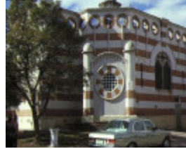
1 methodist church cnr deakin avenue & tenth street mildura side view
