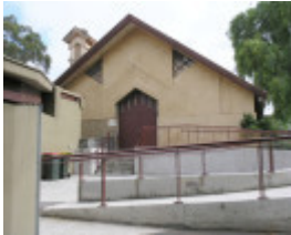
ESSENDON INCINERATOR COMPLEX SOHE 2008
