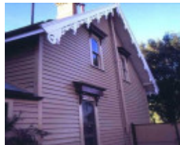
h00139 the american cottage station st coburg side view
