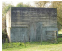
Concrete silage store from west 2017.jpg
