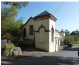
dairy factory from sth east 2017.jpg
