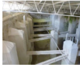
Tunnel from north 2017.jpg
