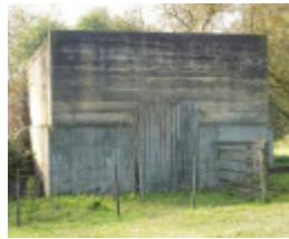
Concrete silage store from west 2017.jpg
