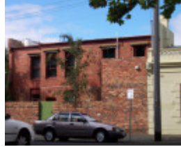
Rear of 366 Rathdowne Street.JPG
