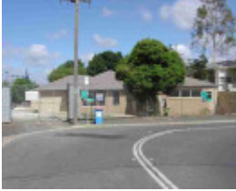
richmond waltham street richmond waltham street 44
