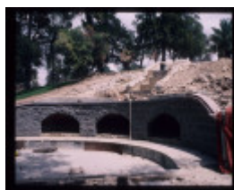
FORMER GOVERNMENT CAMP PRECINCT (ROSALIND PARK) EXCAVATION
