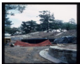
FORMER GOVERNMENT CAMP PRECINCT (ROSALIND PARK) EXCAVATION
