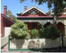
carlton north park street carlton north park street 446
