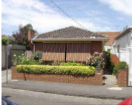
richmond miller street richmond miller street 1
