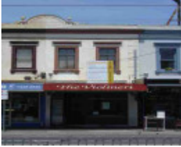
burnley bridge road burnley bridge road 500
