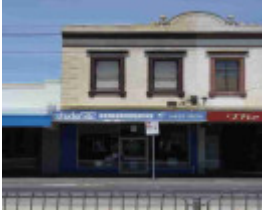
burnley bridge road burnley bridge road 502
