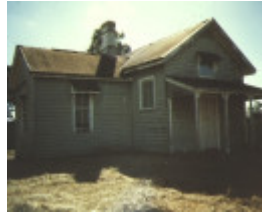
balmoral court house glendinging street balmoral front elevation feb1986
