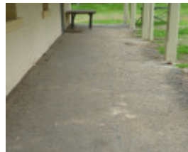
Before Photograph - Reference F3875 2014
