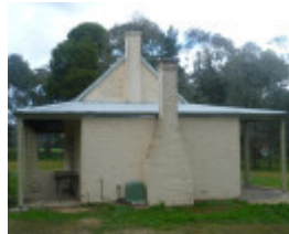
Before Photograph - Reference F3875 2014
