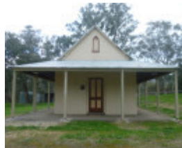
Before Photograph - Reference F3875 2014
