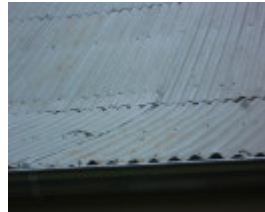
Before Photograph - Reference F3875 2014
