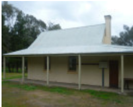
Before Photograph - Reference F3875 2014
