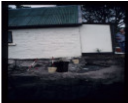
LIMESTONE COTTAGE EXCAVATION
