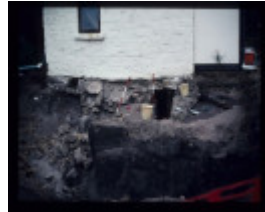
LIMESTONE COTTAGE EXCAVATION
