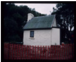
LIMESTONE COTTAGE EXCAVATION
