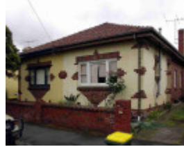
Richmond Charlotte Street 13-15.JPG
