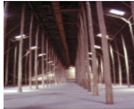
murtoa grain store wimmera hwy murtoa interior from ground view
