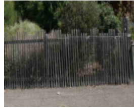
Fence - 123-125 Arnold Street
